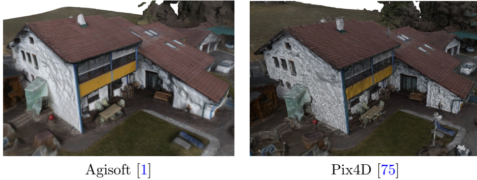
Figure 6.6: Results from commercial reconstruction pipelines of the House dataset. Compared to the reconstruction of the proposed approach (see Figure 6.26), Agisoft and Pix4D do not generate planar surfaces and straight edges, as they use no shape or semantic priors. The façades and roofs are noisy and some scene parts are smoothed too much and become rounded (e.g., building edges, chimney).
