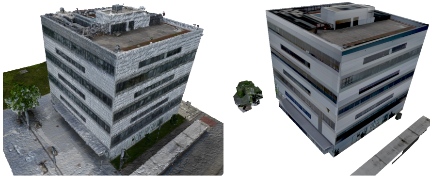
Figure 4.1: Meshed dense 3D reconstruction and resulting regularized model. Left: A 3D building reconstruction created from aerial images taken by an Unmanned Aerial Vehicle (UAV) . The camera poses and initial 3D structure were computed with SfM , then a dense model was computed with Sure [79] which was finally meshed using Poisson surface reconstruction [43] (visualized with vertex coloring). Such a mesh can be used as input for our approach. Right: Resulting regularized model from our pipeline, textured with [93]. We deliver clean and smooth surfaces whereas the meshed dense point cloud contains a lot of noise.
