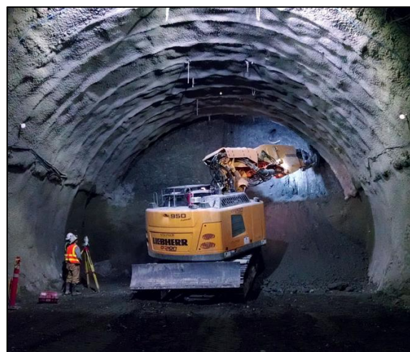
Figure 49: Excavation, shotcreting and monitoring according to the NATM [33]
