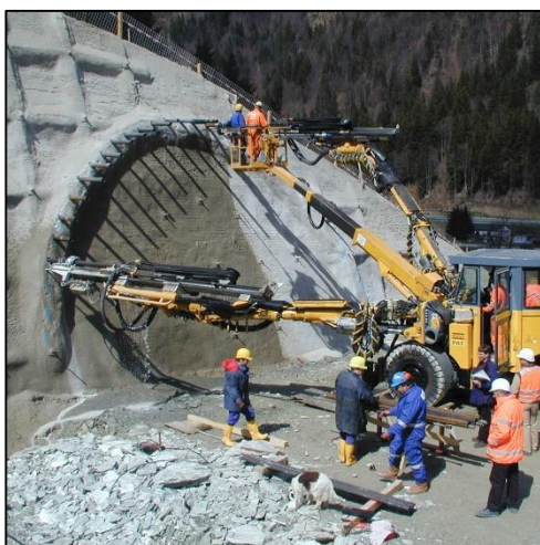
Figure 48: Construction of a pipe Umbrella [32]
