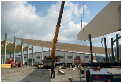
Fig. 1 Assembly of a roof structure with fish belly beam
