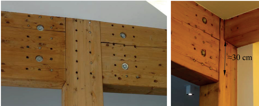
Fig. 5 Appearance of shrinkage cracks in the area of a flitch plate dowel - rigid connection in very dry conditions
