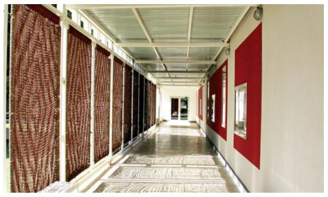
Fig. 2: A detail of the porticos of the Salam Centre with the twined vegetal panels on the left and the small double-screen windows on the right (photo by *Emergency*  $NGO^6$ )
