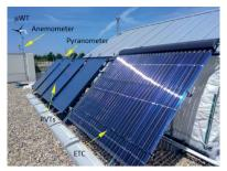
Figure 2.1: Detail of the  $\mu$ WT, PVTs and ETC of the pilot unit.
