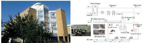
Figure 1: Building enclosure, heating and ventilation scheme of the EES Q Building Testbed at KTH.
