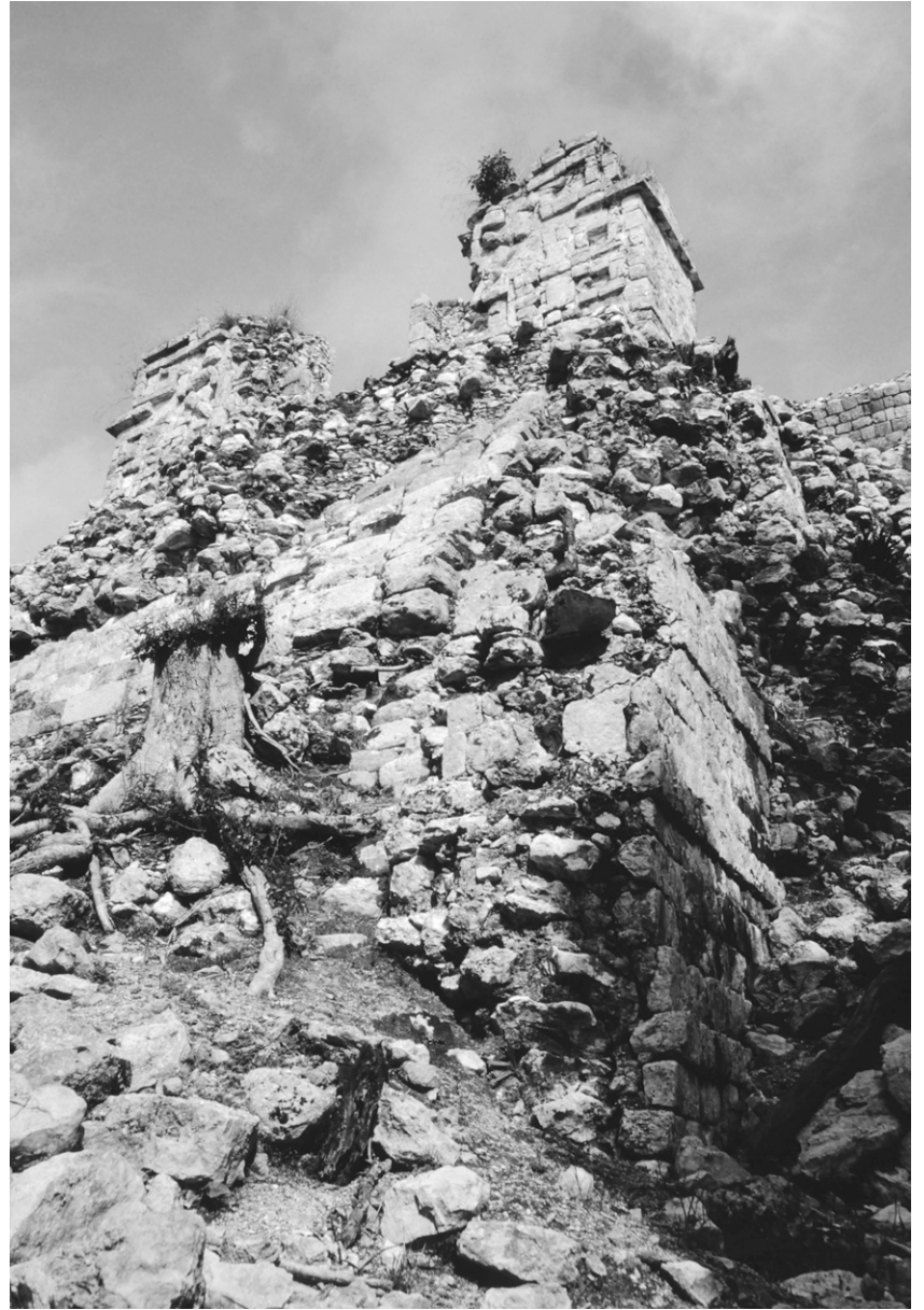
Fig. 107 The situation in 2001 before reconstruction shows that the mega steps do not reach the breadth of the earlier stairway. There must have been something in-between – possibly a recessing ramp. Photograph: H. Hohmann 2001
