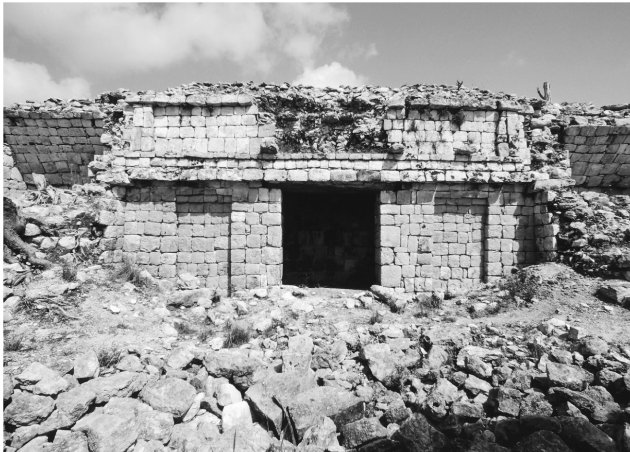
Fig. 98 The eastern façade of Room 42, the quite large, representative and most central room of the Palace on the third floor was quite well preserved. It shows the entrance and two pseudo side entrances. Photograph: H. Hohmann 2001
