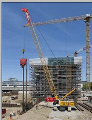
Crawler crane – LR 1100
