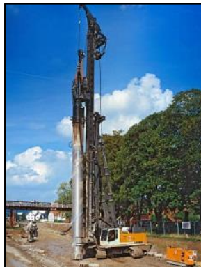
Piling & drilling rig LRB 255
