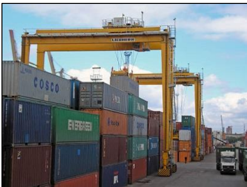
Rubber tyred gantry cranes
