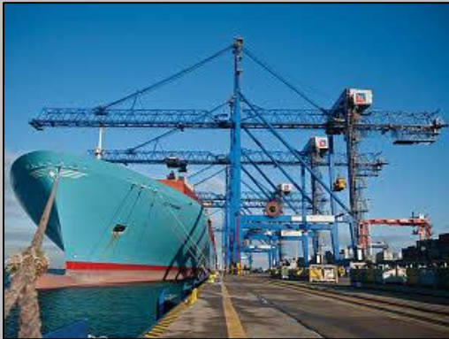
Rail-mounted ship-to-shore container cranes
