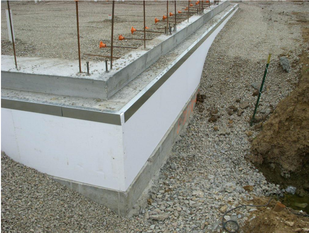
Figure 7. EPS boards on basement walls (breastultrasound.org)
