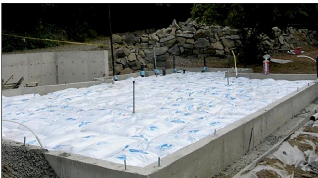
Figure 21. Perlite bags tightly placed on grade
