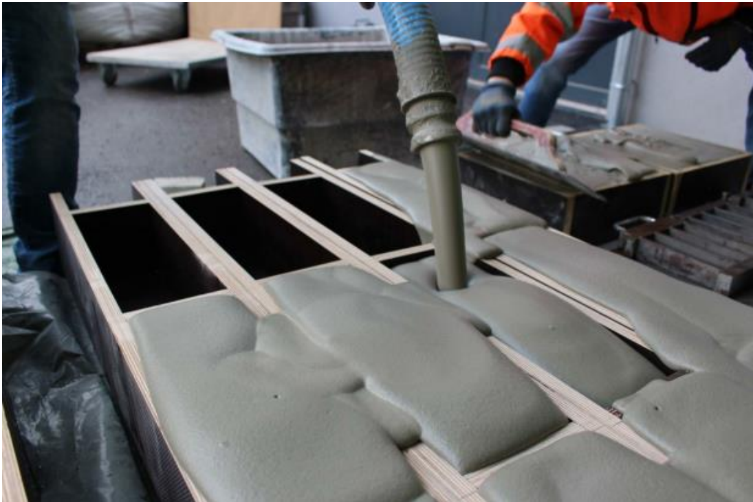
Figure 31. Foam concrete panels preparation
