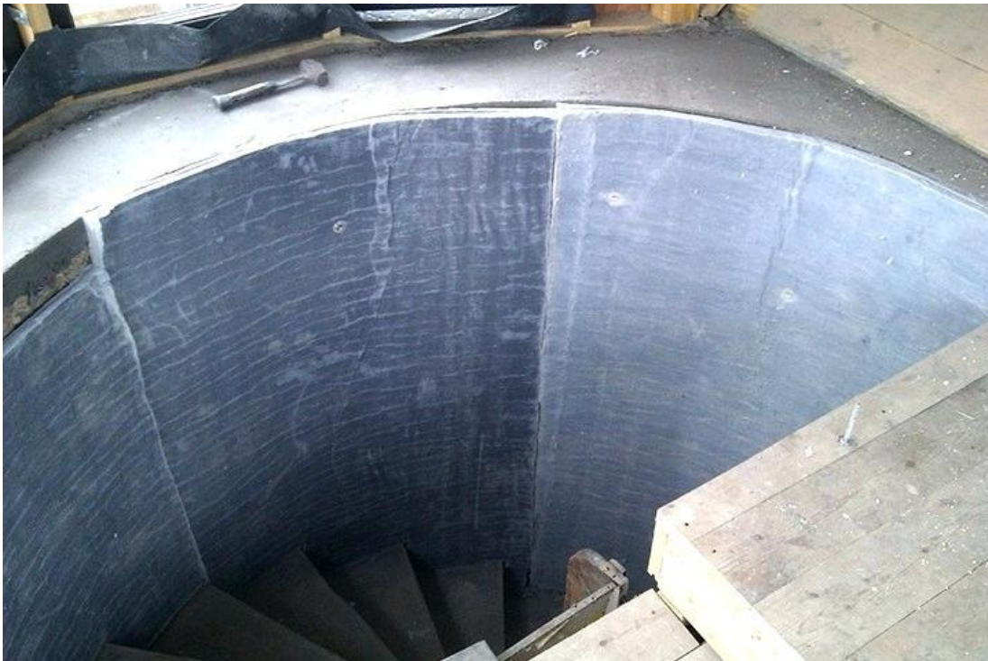
Figure 12. Silica Aerogel foundation stairwell (mipsbe)
