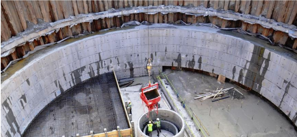
Figure 55: Avonspark Street segmented Shaft Installation
