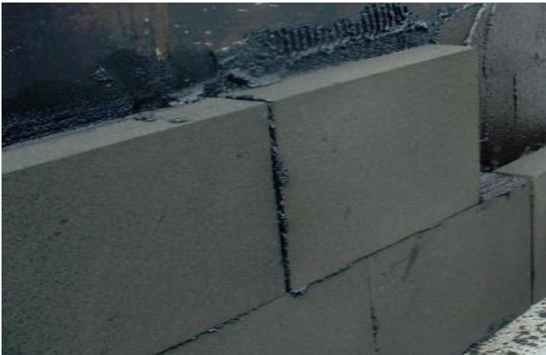
Figure 28. Foam glass board installation on basement walls (BuildingGreen)
