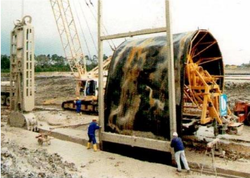
Figure 63 : Installation of plastic liner sheet in D-Wall, Central Waste Dump, Huenxe
