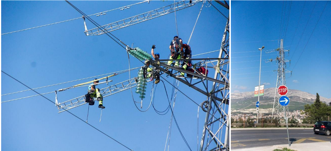
Figure 7.6 – Reconductoring project on OHL 110 kV Vrboran - Dujmovača (HOPS, Croatia).
