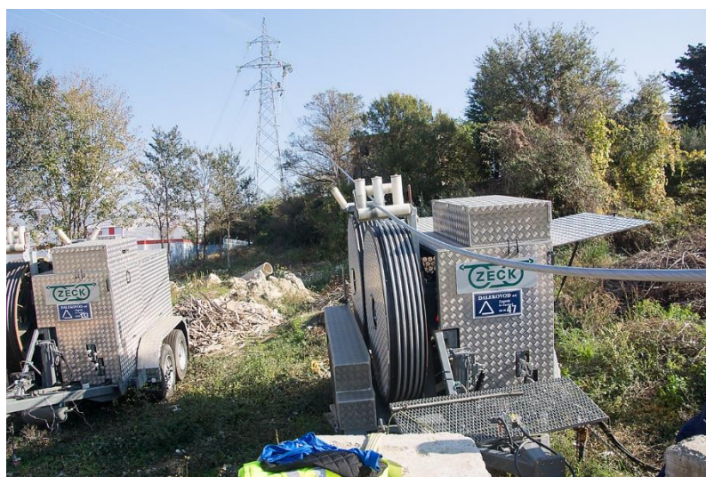
Figure 7.5 – Reconductoring project on OHL 110 kV Vrboran - Dujmovača (HOPS, Croatia).
