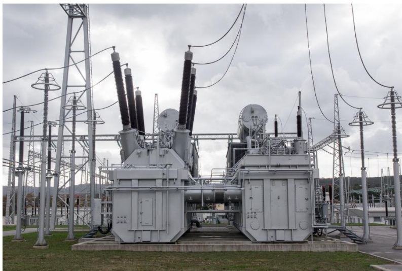
Figure 6.5 – Two-tank design, PST in SS Divača (ELES, Slovenia)
