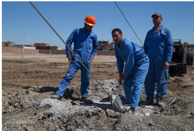
Figure 30: Hoisting the mast with a manual grip hoist
