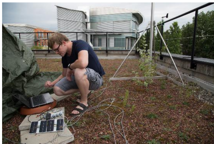
Figure 19: Testing of system supply and measuring data in Graz with electronic specialist Martin Mauernböck
