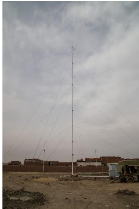
Figure 33: The final wind mast position in operation
