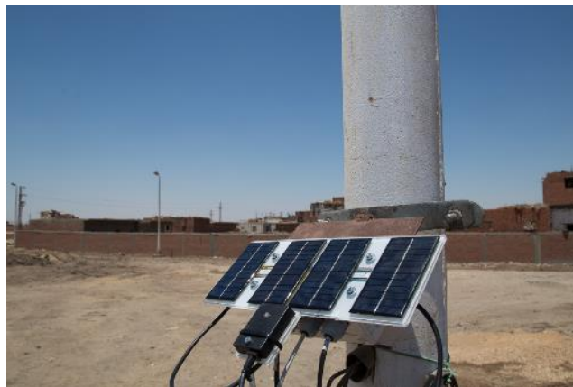
Figure 21: The final data logger on the mast after its installation
