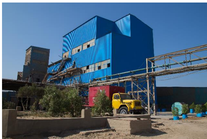
Figure 37: Emisal Anlage Sept. 2018
