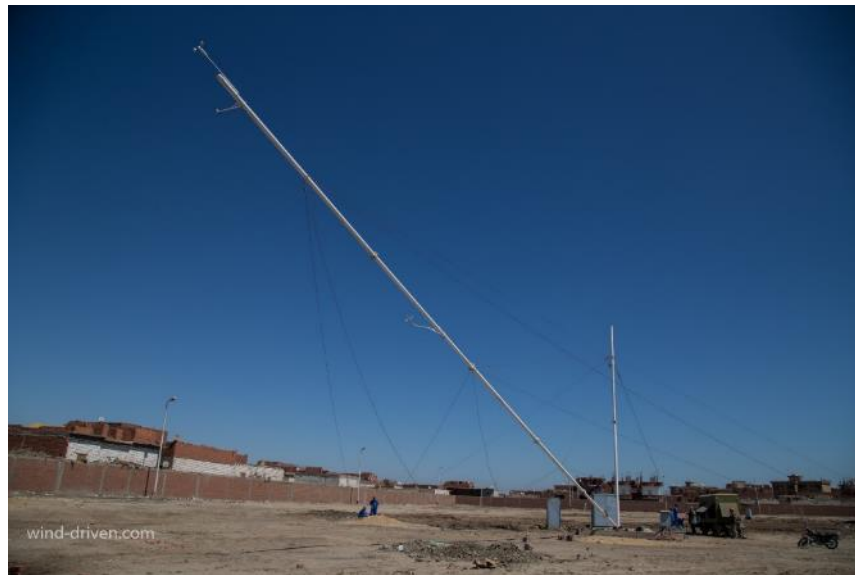
Figure 31: 30m wind pole during erection phase
