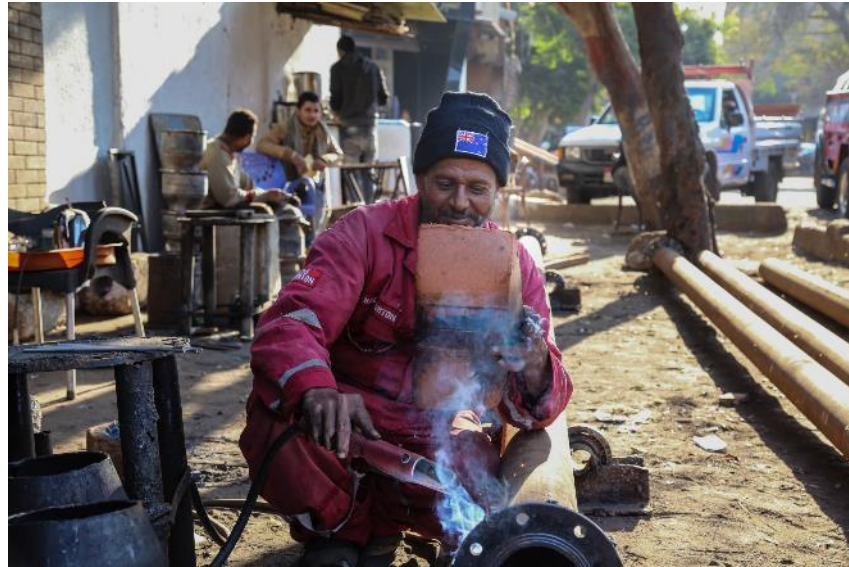
Figure 24: Welding the flanges for the mast, in eastern part of Cairo
