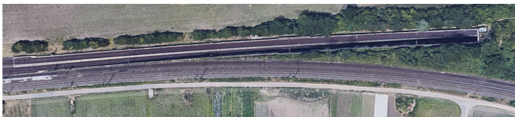
Figure 1.8: The part of the track outside the tunnel runs parallel to a second track. In this part also trains of the neighbour track can be measured by the system.
