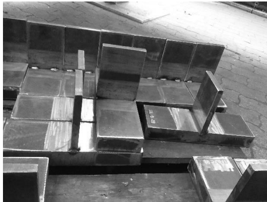
Fig. 1 Tack welded T-joints before welding.
