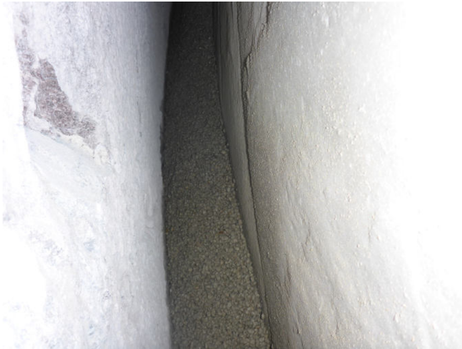
Figure 57: Image of the pea gravel slope within the annular gap behind the shield tail. View against the advance direction (taken from Henzinger et al., 2018).
