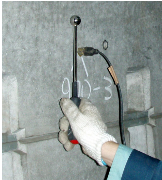
Figure 14: Illustration of the impact-echo method. Impactor (metal sphere) with a diameter of 25 mm close to sensor (taken from Aggelis et al., 2008).
