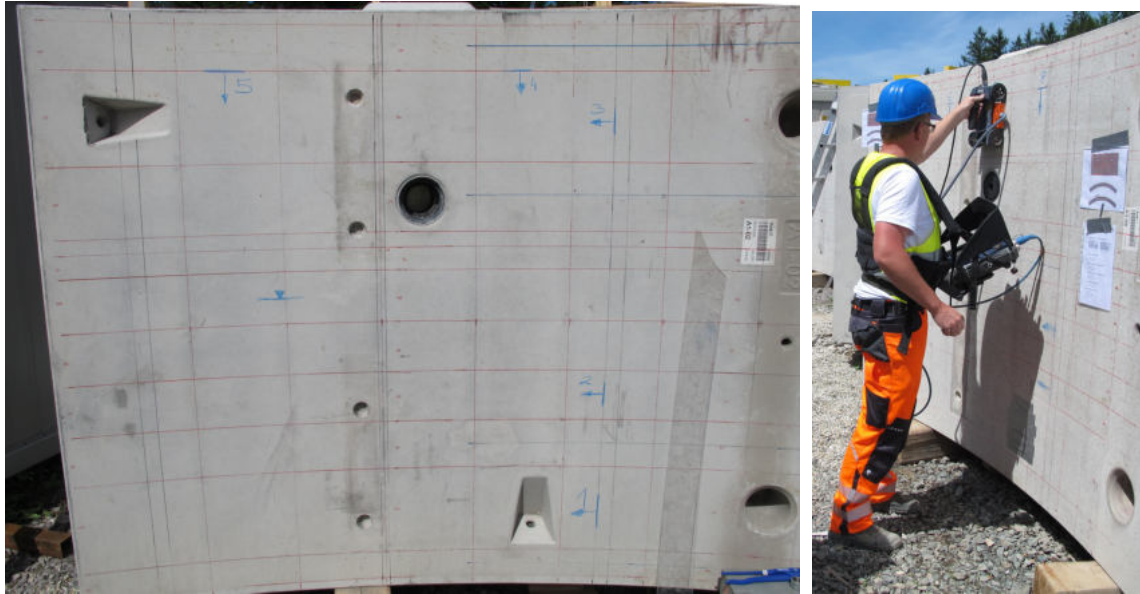
(a) Reinforcement plan (red) and measuring concept (blue) illustrated on the inner surface of the segment type A. (b) GPR measurements with the “SIR 4000” handheld device.
