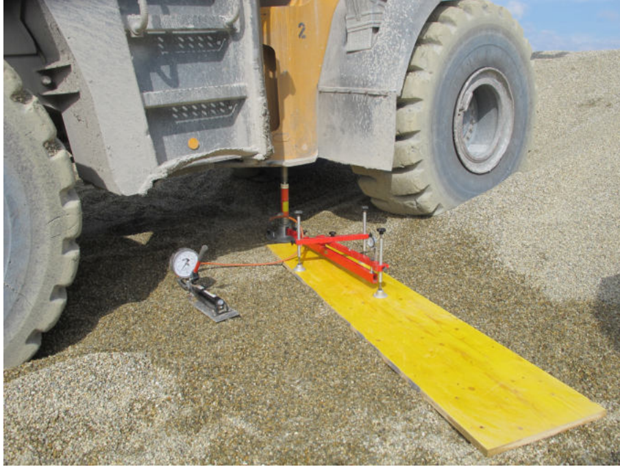
Figure 27: Load plate test on pea gravel.
