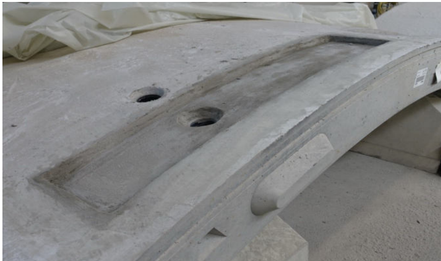
Figure 71: Notch for the geotextile tube on the exterior surface of one segment (taken from Henzinger et al., 2018).
