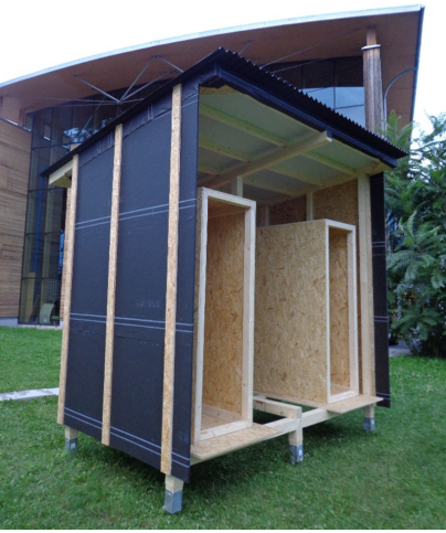
FIGURE 8-3: COMPLETED SHELTER WITH THE TWO BOXES
