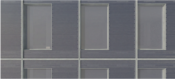
FIGURE 4-13 SOLAR COLLECTOR SANDWICH PANELS WITH VISIBLE PIPEWORK AND ANTI-REFLECTION COATING FOR SURFACE GLASS [2]
