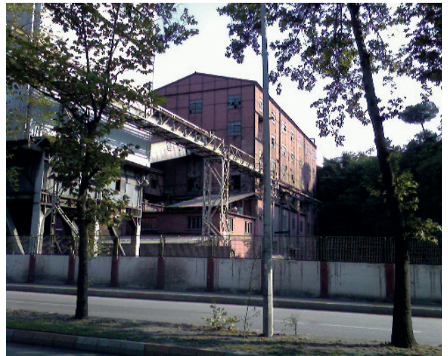
[Figure 105] (right below) conveyors towards port area above the road. Separation and isolation with walls.
