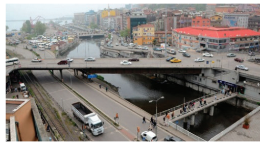
[Figure 88] Overview of Zonguldak Fevkani Bridge, cantilevered bridge.
