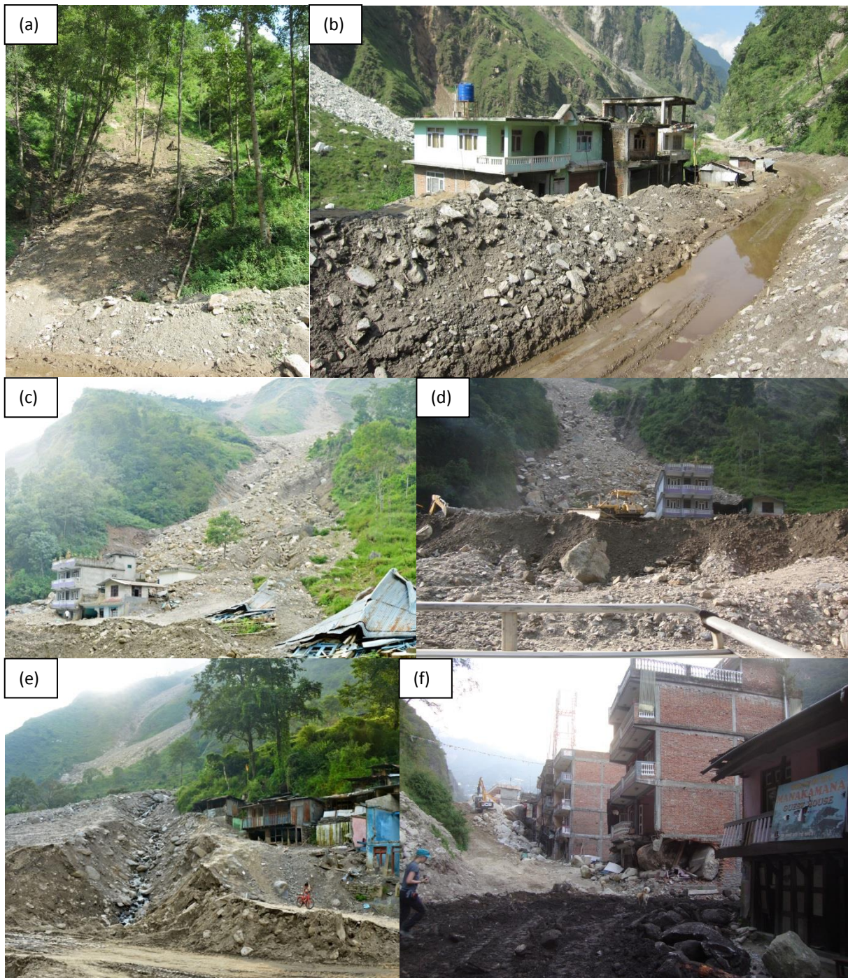
Fig. 64: Landslides triggered by the earthquake and activated by the monsoon at Araniko Highway. (a) source area first landslide; (b) deposit area first landslide, blocked road (reopened on picture) and destroyed houses; (c) and (d) second landslide source and deposit area, blocked road and destroyed buildings, bulldozer marks former road; (e) parts of third landslide (front) and source area of second landslide (background); (f) fourth landslide in Kodari, destroying buildings and blocking road for several months.
