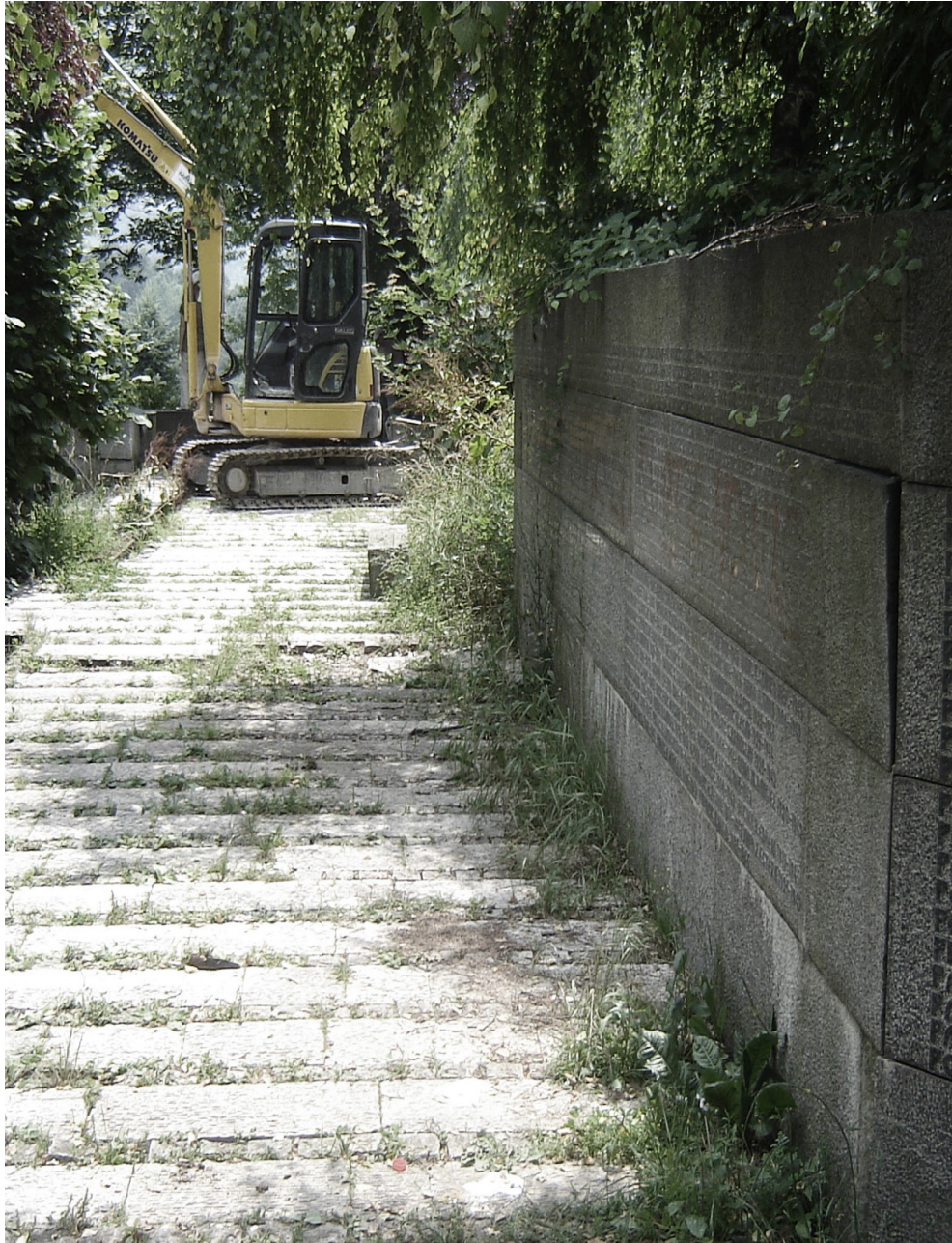
42. First stage of renovation and reconstruction, 2010
