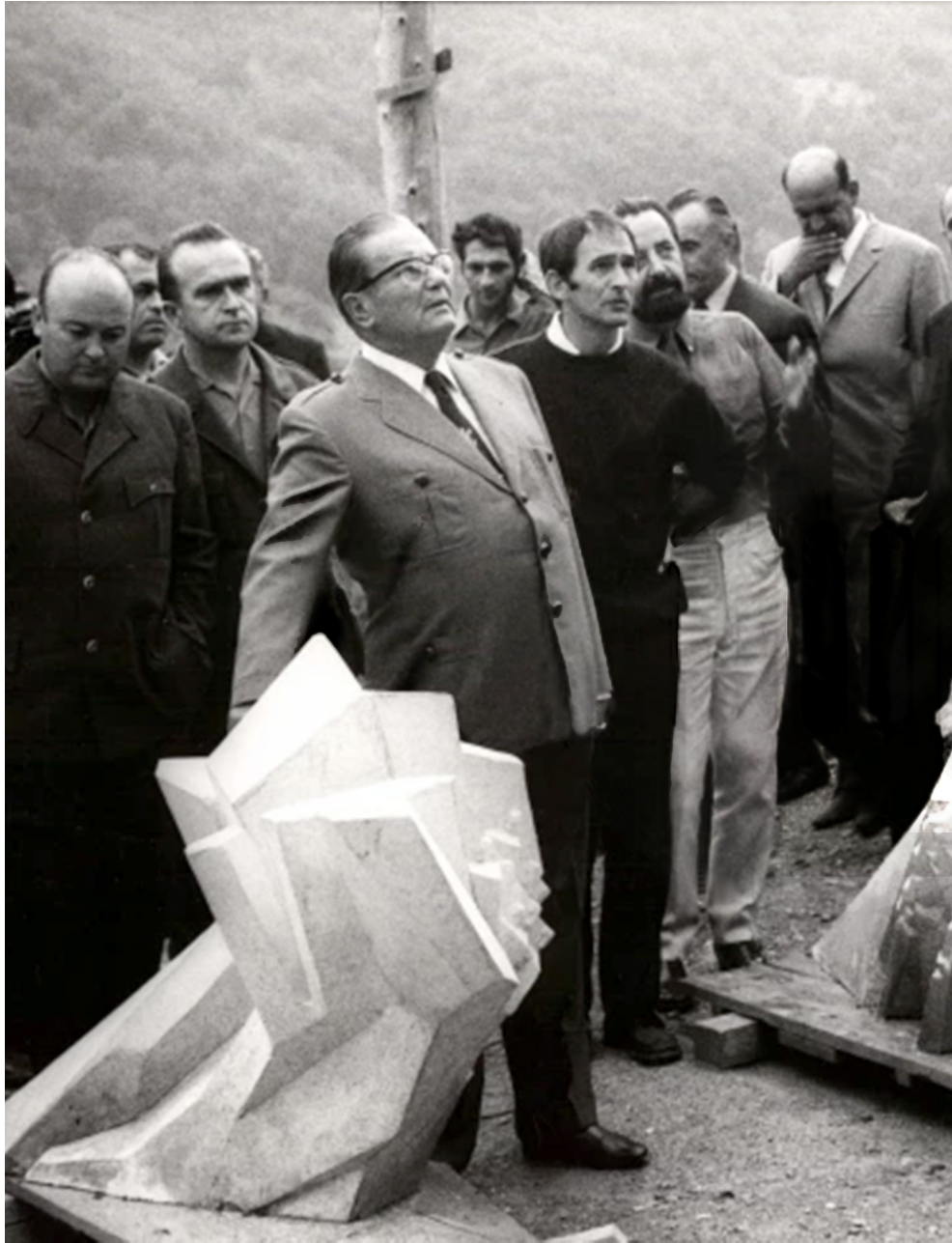
9. Construction of the Tjentište memorial complex during Josip Broz Tito's visit, late 1960s
