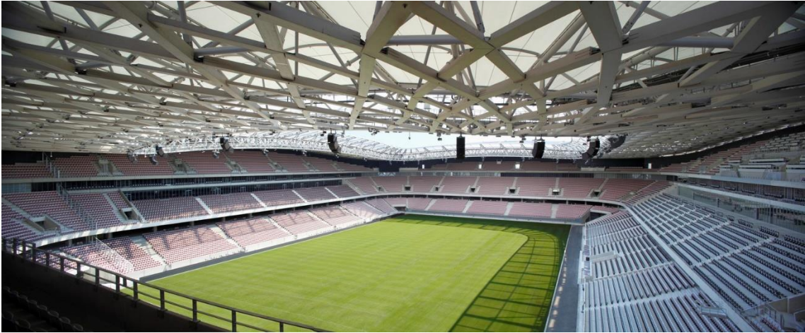
Fig9. Willemote Allianz Riviera, roof structure
