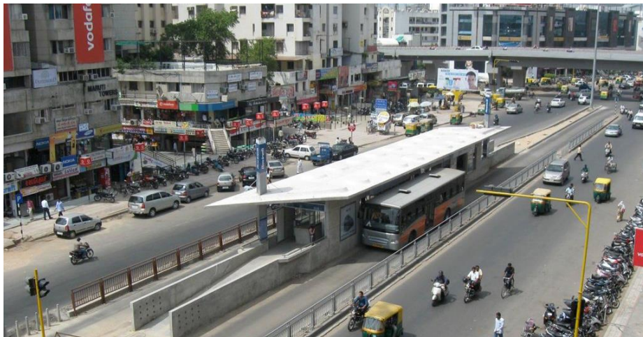
Figure 65: BRT system in Ahmedabad [ITPD, 2015]
