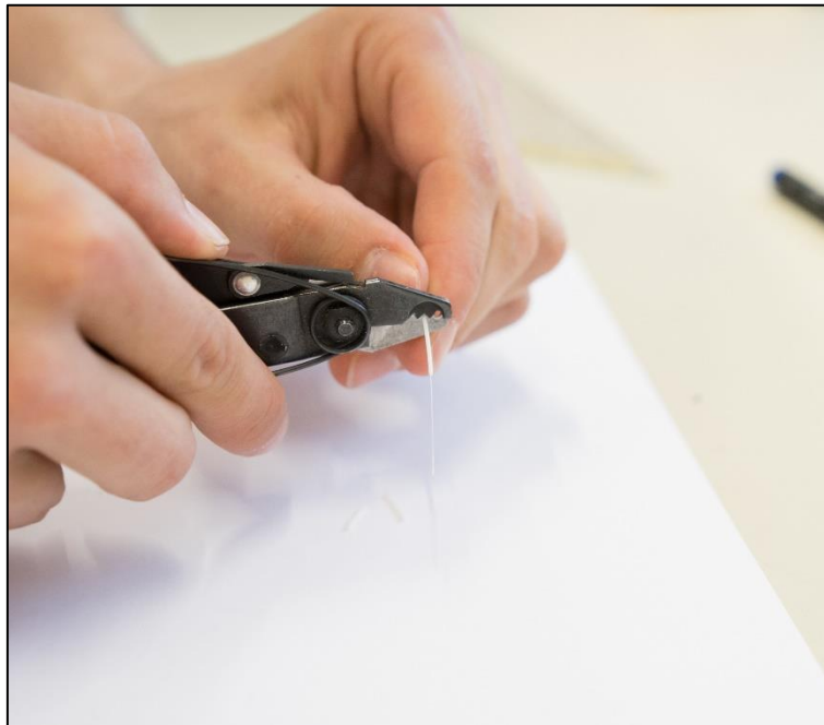
Figure 5-10: Removing the coating from the optical fiber for splicing purpose
