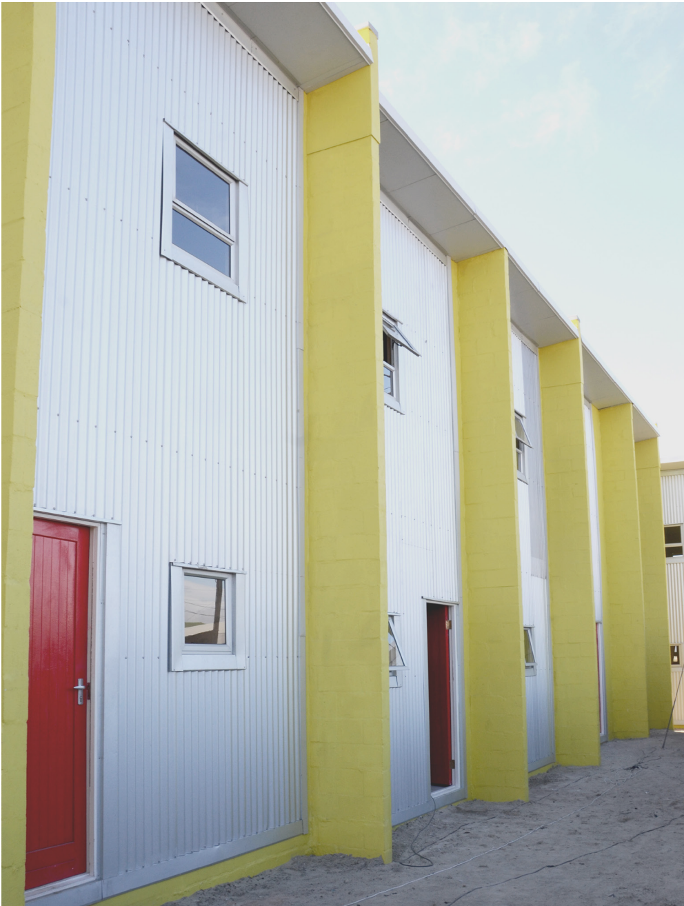
Figure 4.10 Empower Shack Phase two, BT North, completed in 2018
