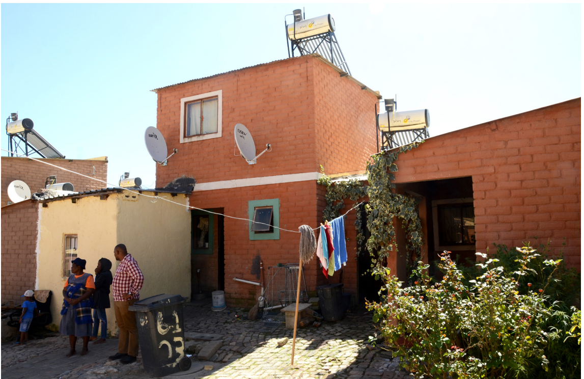
Figure 2.8 RDP houses in Alexandra Ext. 9 with extension built by the resident
