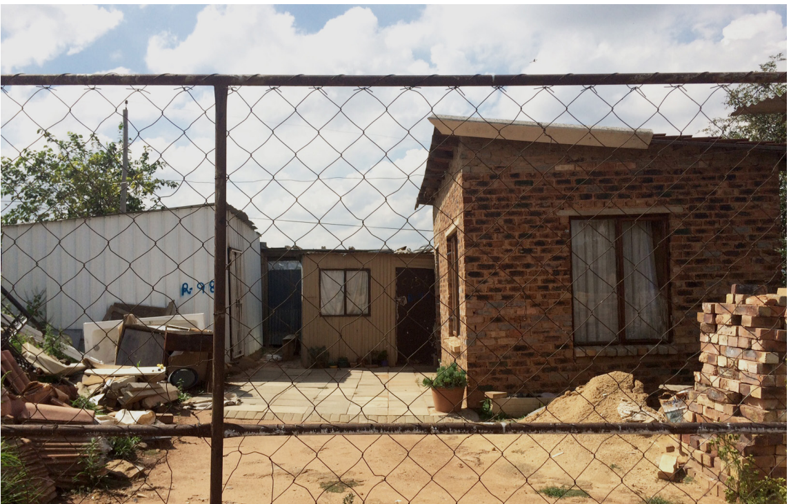
Figure 3.12 Upgraded shack with additional structures in corrugated iron and brick
