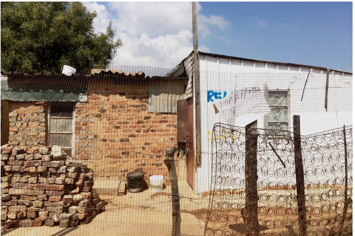
Figure 3.1 Ruimsig upgraded shack with brick extension by resident
