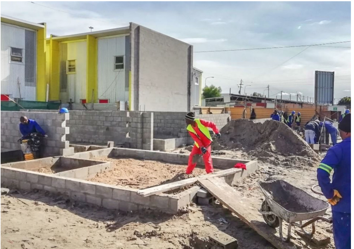
Figure 4.1 Empower Shack phase two under construction
