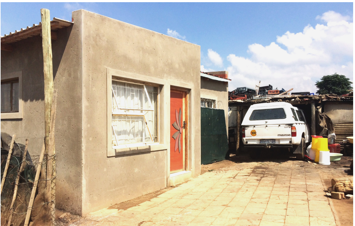
Figure 3.10 House completely rebuilt by resident, in plastered brick
