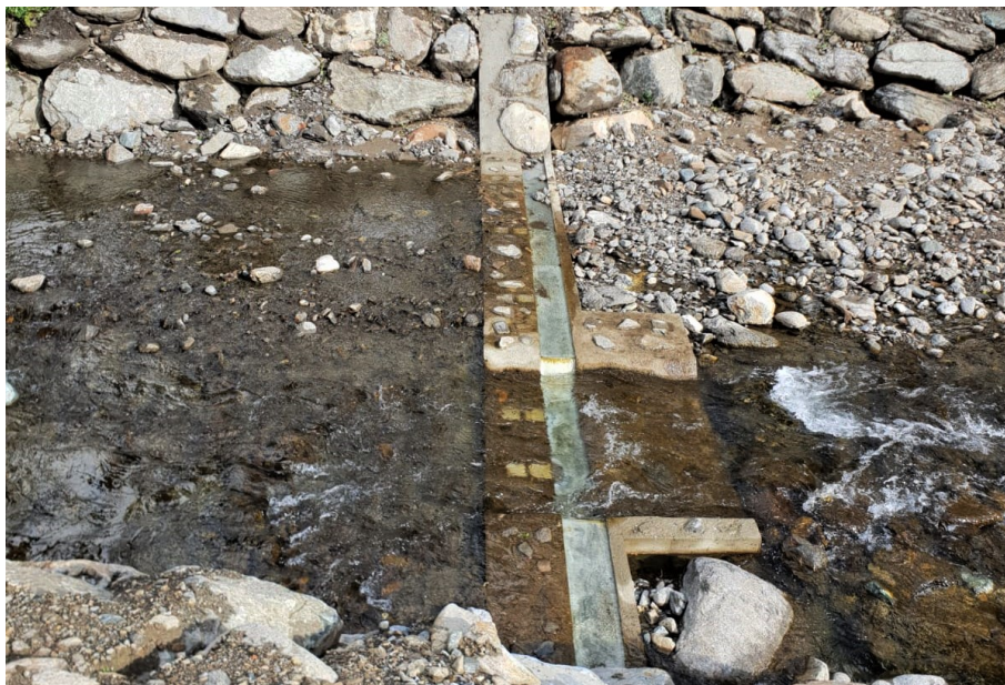
Figure 4.15: Back-filled and finished submerged weir
