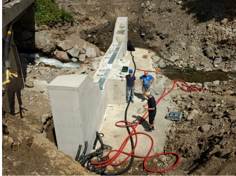
Figure 4.14: Submerged weir under construction July 2018
