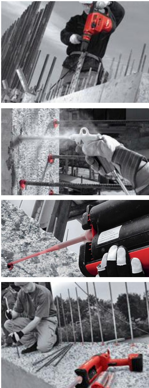
Figure 3. Post-installed fastening systems (drilling, cleaning, injection, setting); taken from reference 8.
