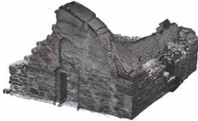
Figure 2.4: Medium density, colored point cloud of the St. Petka Church from Raykovska, Bevan, and Vasiliev (2015)
