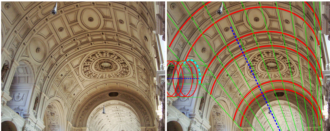
Figure 3.3.: Another example of arches of a church (left). Two possible setups for coordinate systems (right) are highlighted - there is the main one, and a smaller side one on the left. Colors are chosen as in Figure 3.2. The dashed light blue line depicts the line where both coordinate systems intersect. Having both coordinate systems available allows for the exact generation of the line and geometry on it. Image taken from [2].
