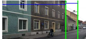
(h) Found corners (green) and defined facades (blue) shown over the rectified input image.
