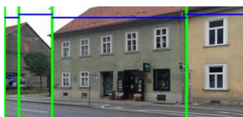
(h) Found corners (green) and defined facades (blue) shown over the rectified input image.
