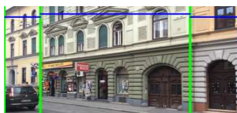
(h) Found corners (green) and defined facades (blue) shown over the rectified input image.
