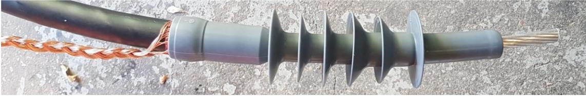
Figure 6-4: Installed double standard 12/20 kV AC cable termination
