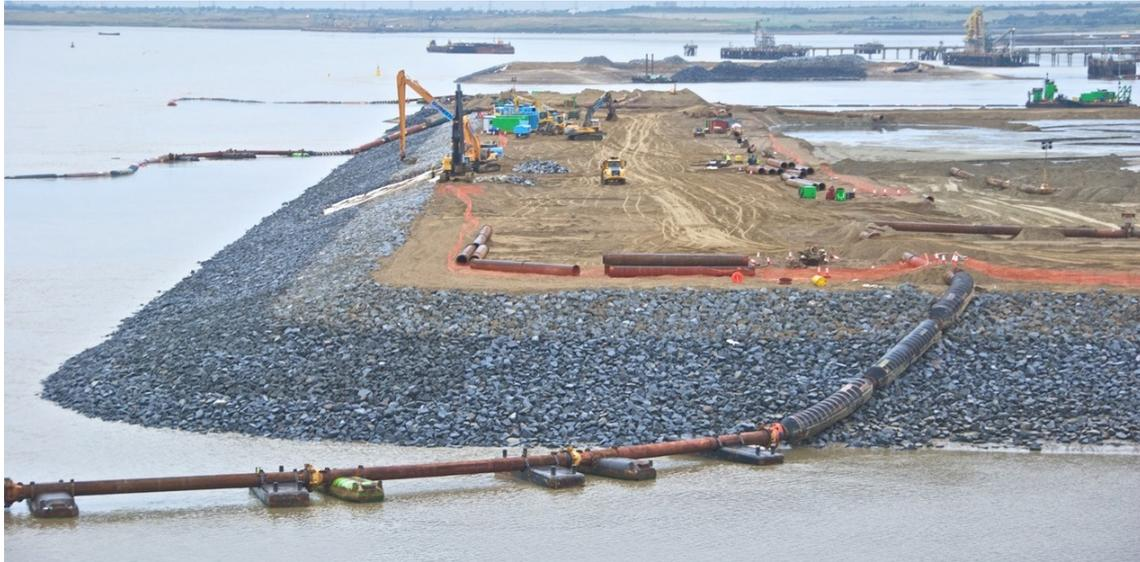
Fig. 7: Transition between floating and onshore pipeline [12]
