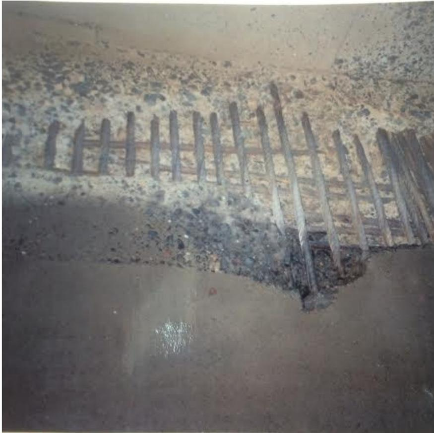
Fig. 1 Prototype photograph showing exposed reinforcement inside Tunnel due to cavitations
