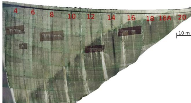
The resulting textured 3D surface models (Fig. 2) and ortho images achieve a comprehensive documentation of the downstream side of the dam. Detect or already known defects are acquired with high-resolution automatically. The location (coordinates) and appearance (photos) of the defects are documented and thus changes on the concrete surface are automatically identified and quantified.
