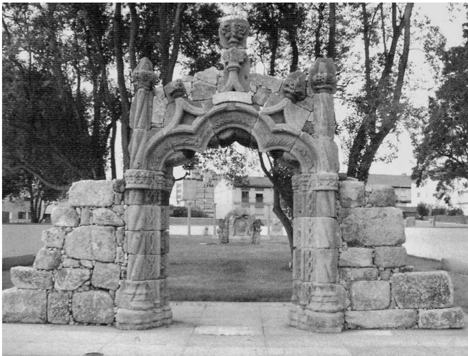
Fig. 5. Manelino portico (1983). Historical Archive. Porto City Hall.
