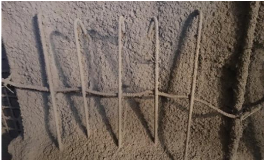
Figure 7.4: Installation of the connecting element at Tunnel Stein.
