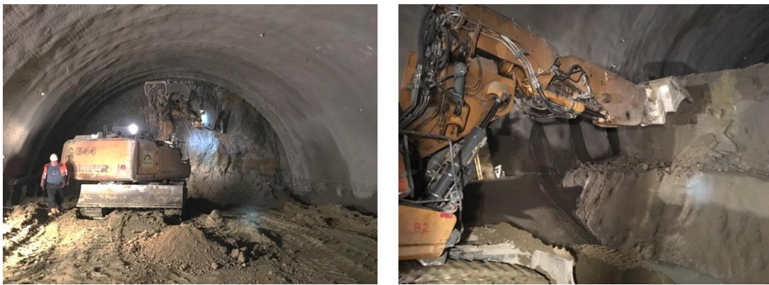
Figure 7.1: Top heading-bench excavation of the Tunnel Stein.
