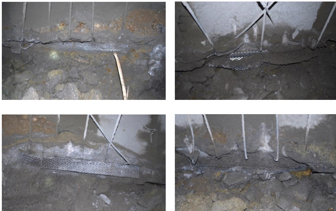
(a) Intended execution of the exposure of the connecting element.
