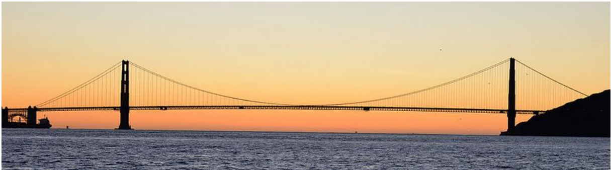
Abbildung 1 Golden Gate Bridge in San Francisco [1]
