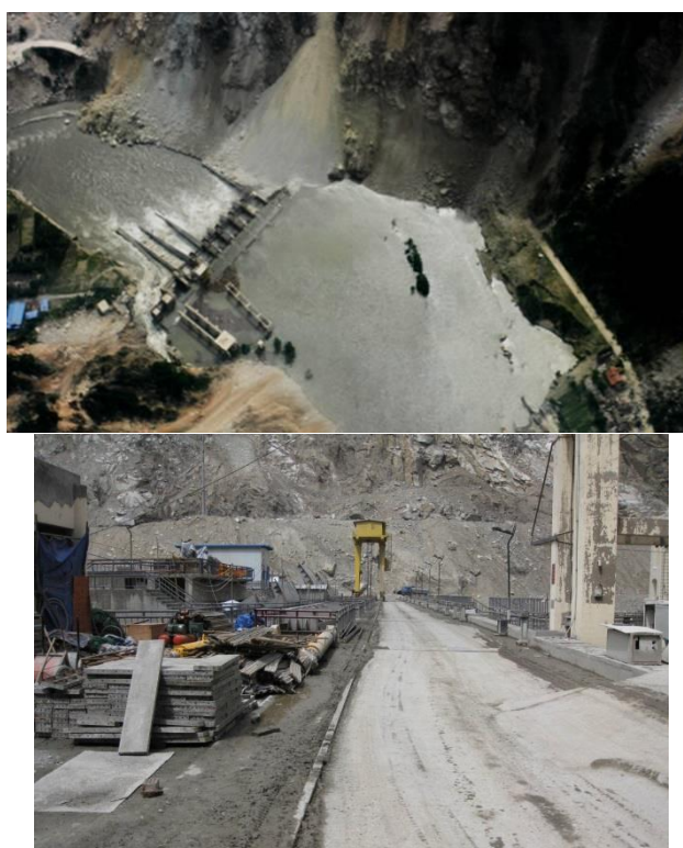
Figure 1. Overtopping of run-of-river power plant due to failure of gate operation (left) and mud deposited on crest of overtopped run-of-river power plant (right) (Wenchuan earthquake in China)
