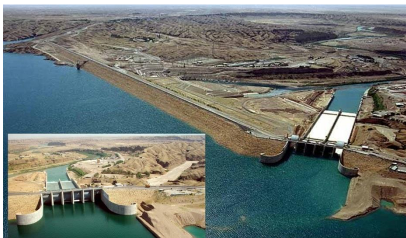
Figure 1- An example of the use of gated spillways with radial gates as a flood discharge system at the sideway of Karkheh dam in Khuzestan province in Iran.
