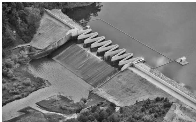
**Figure 1: Example of a labyrinth weir (after Crookston and Tullis, 2013)**
