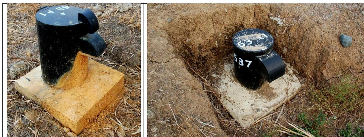
**Figure 10: Daule Peripa reservoir rim dike, relief wells showing erosion and settlement cracks.**
