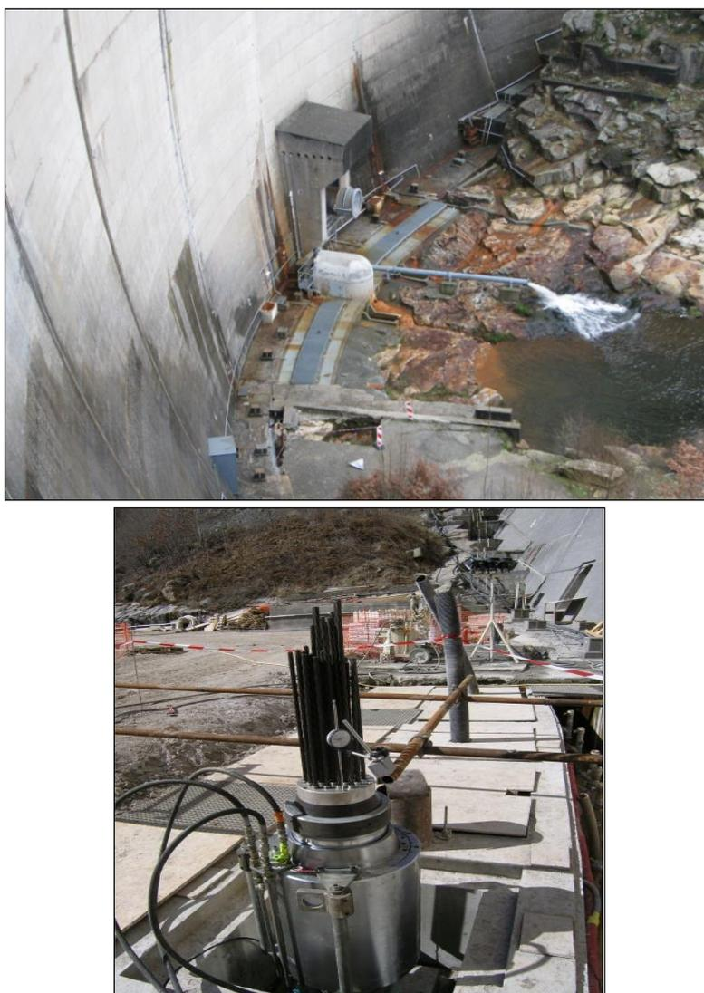
**Figure 6 view of the downstream beam and of the installation of the anchors.**
