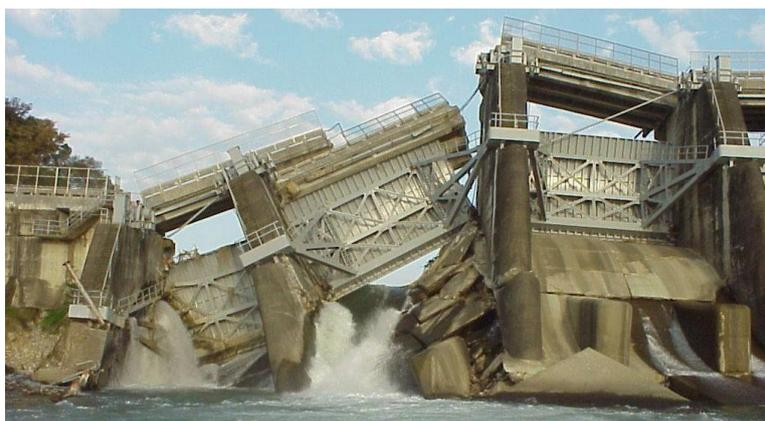
**Figure 2: Failure of two bays of the Shih-Kang weir caused by (mainly vertical) fault movements during the 1999 Chi-Chi earthquake in Taiwan**
