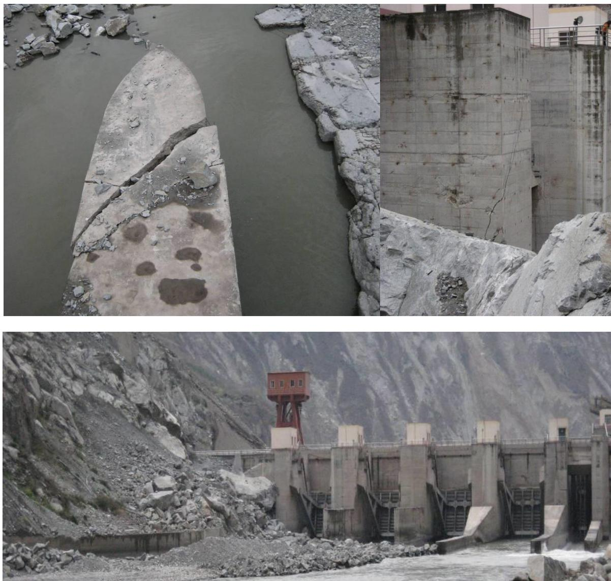
**Figure 3: Damage of spillway piers caused by rockslides during the 2008 Wenchuan earthquake in China**
