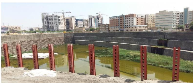
**Figure 3. Water entering the construction sites.**
