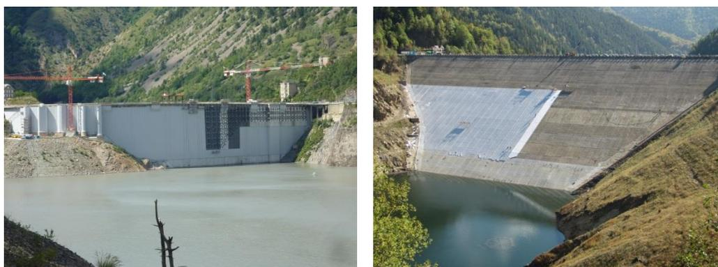
**Figure 2. At left, PVC geocomposite sheets under installation on drainage geonet (the black material on top of the tendons and carbon bands mesh used for structural reinforcement) at Chambon dam in France in 2014. At right, PVC geocomposite sheets under installation on anti-puncture geotextile (the white material) in stage 2 at Pecineagu CFRD in Romania in 2012**
