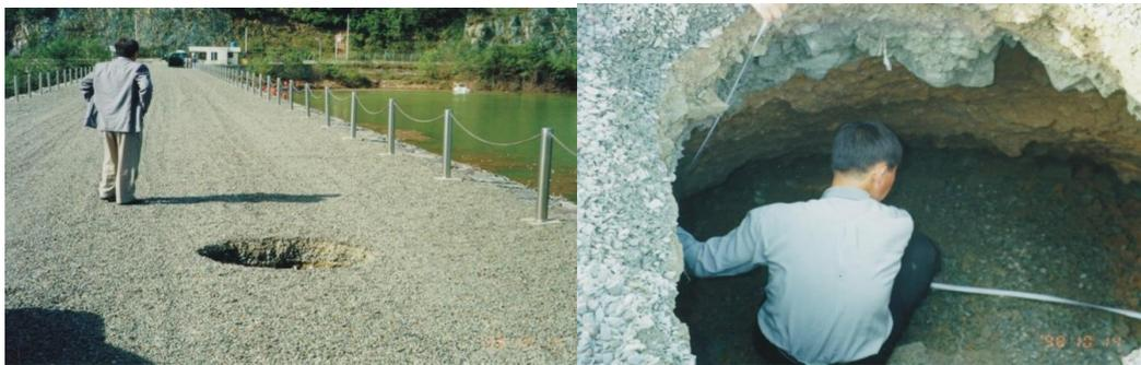
Figure 5. A sinkhole as a consequence of ageing that developed on the crest of the Unmun dam in 1998
