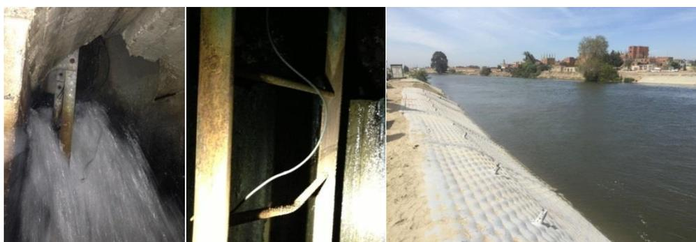
**Figure 5. From left to right, joint 4-5 at Olai dam before and after underwater installation of Carpi external waterstop, and SIBELONMAT<sup>®</sup> installed underwater at Ismailia canal, Egypt 2016**
