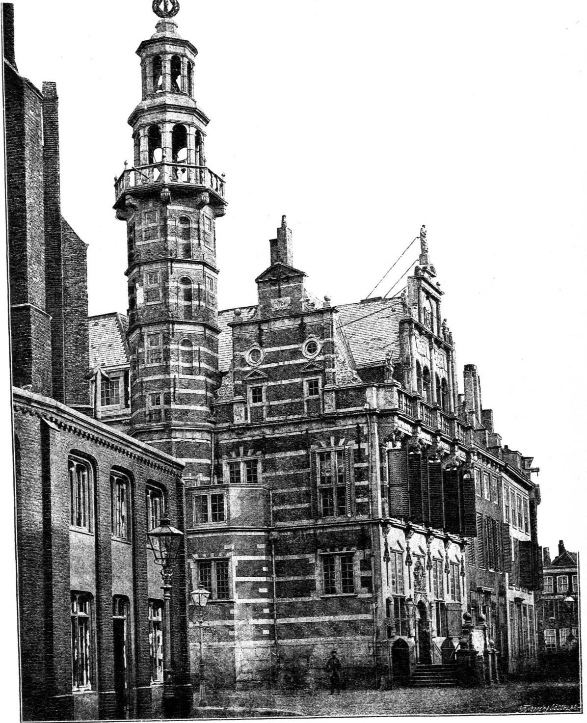
Rathhaus in Haag 90 ).
