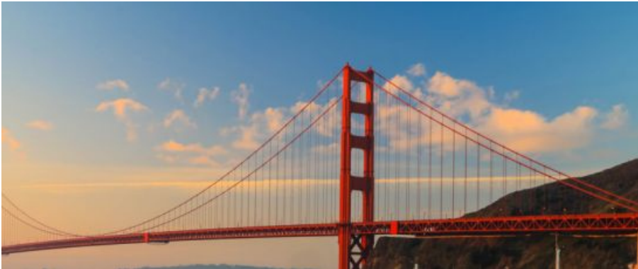
Abbildung 23 Golden Gate Bridge in San Francisco 182
