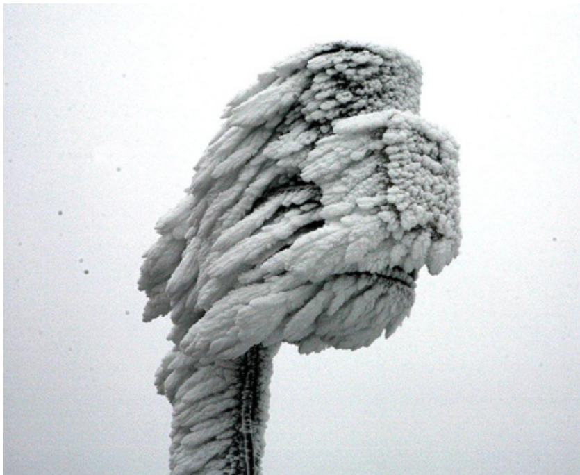
Figure 1.2: Ice covered housing of a rain collector [2].
