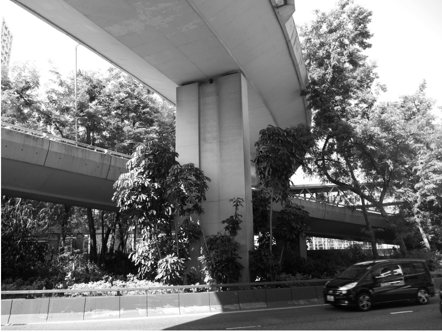
- Motorway — Flyover Intersection, Hung Hom -
