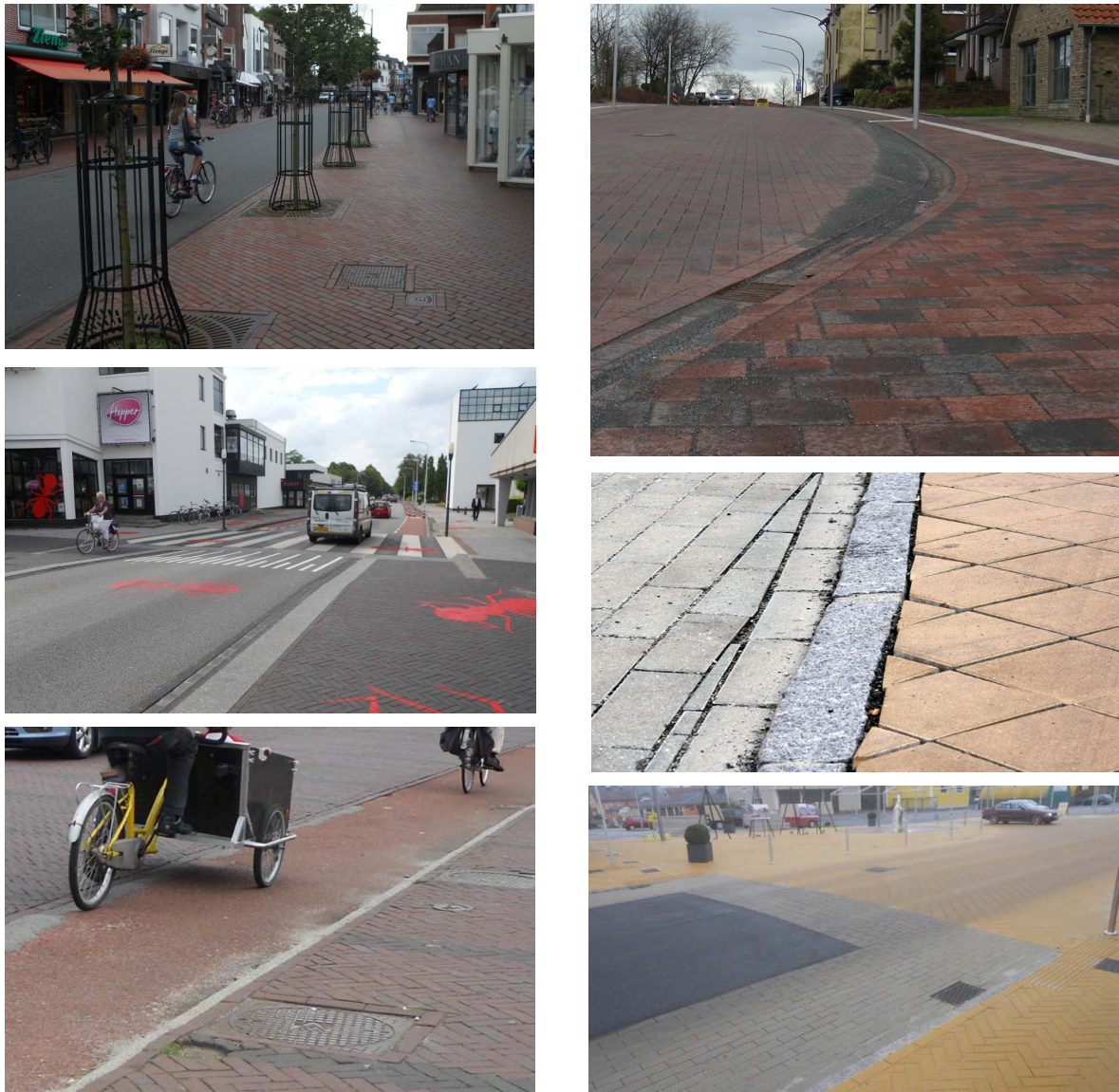
Figure 8.2: Examples of soft segregation of lateral modal designation. Captions from TOP to BOTTOM. LEFT SIDE: Haren (Schönauer, 2009), Drachten (Schönauer, 2009), Haren (Schönauer, 2009). RIGHT SIDE: Bohmte in Germany, (Schönauer, 2009), Gleinstätten in Austria (derstandard.at/blei, 2011), Gleinstätten in Austria (Schönauer, 2009).
