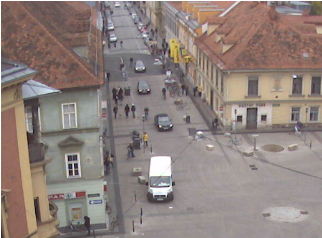
Figure 3.4: Photo of a one-way (for motorized vehicles) road segment leading to the shared space at Sonnenfelsplatz . It illustrates that in the absence of road markings, the boundary of the vehicle's space is constrained by road furniture and bollards.
