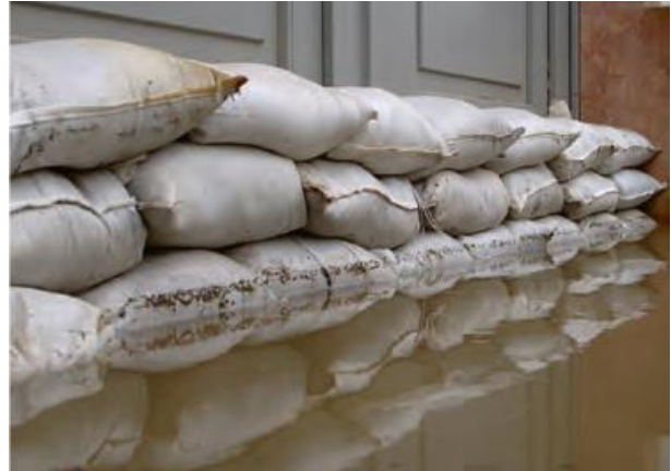
Abb. 40: Sandsackwall [3]
