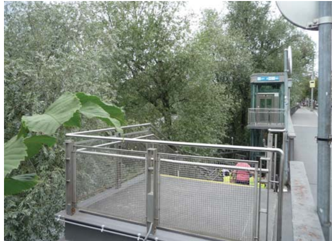
Fig.47 Mur- Insel access | View to staircases and elevator
