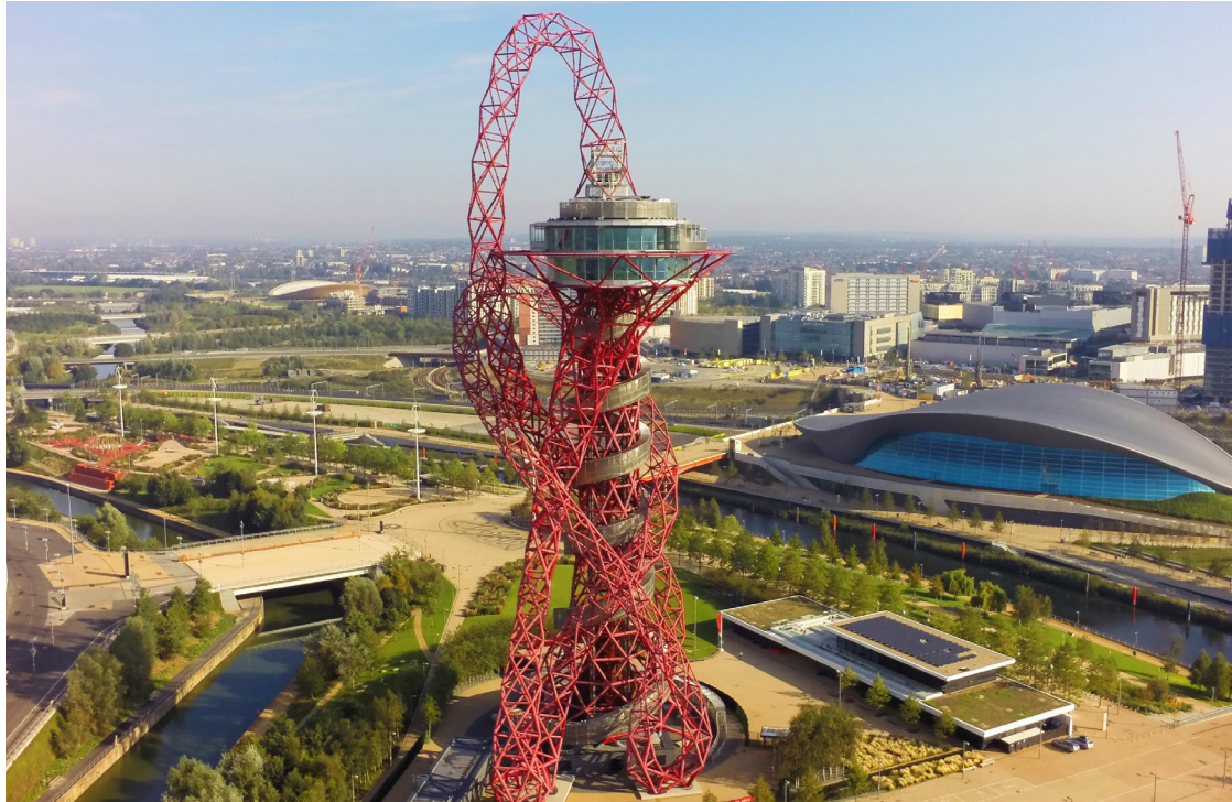
Figure: 41. ArcelorMittal Orbit with Aquatics Center in the Background
