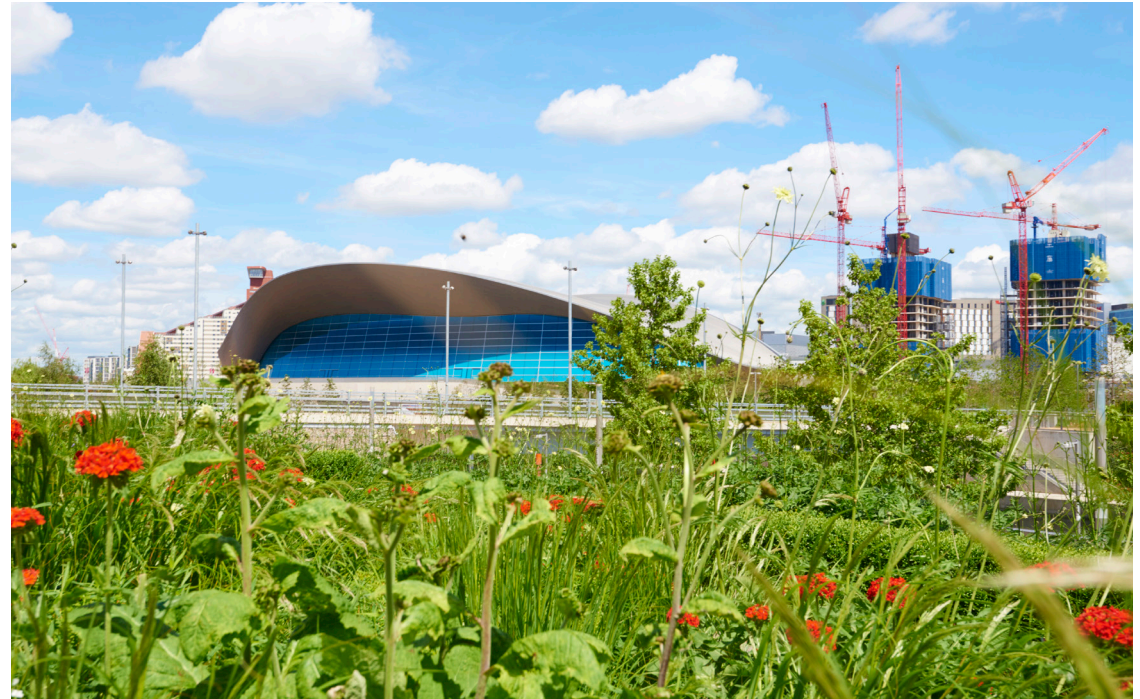
Figure: 23. Aquatics Center with construction work in the background
