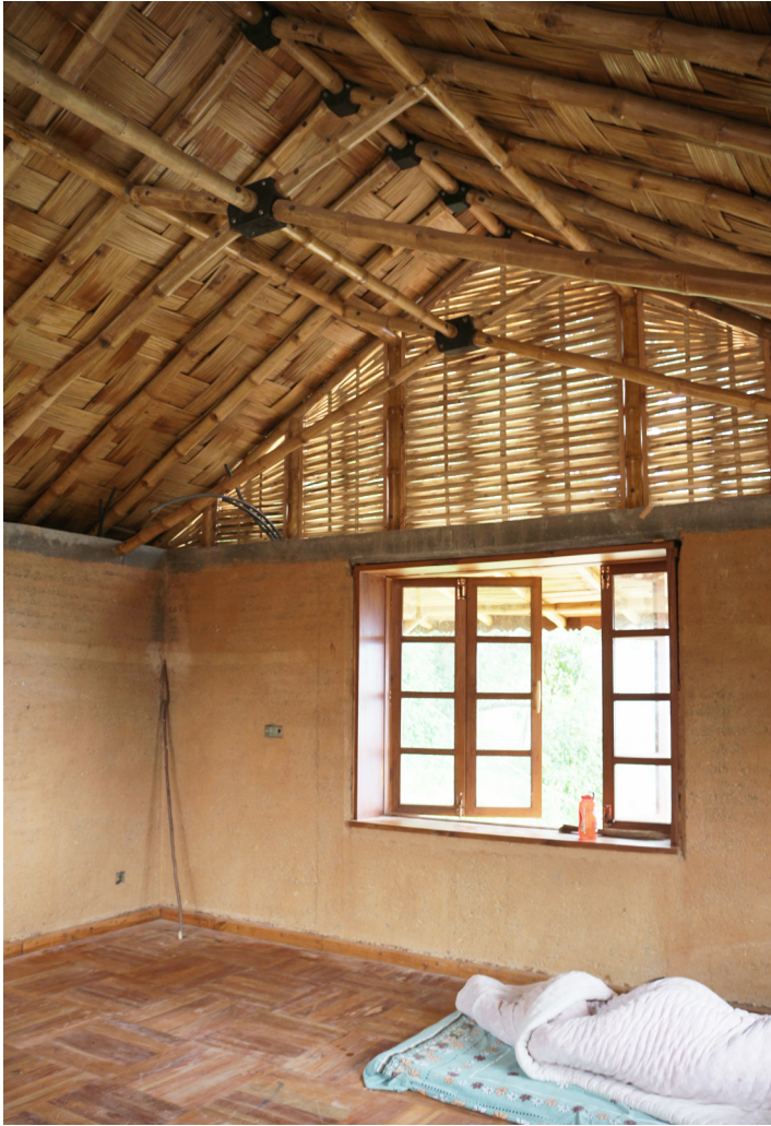
Abb.102: Abari, Dulikhel Learning Center, Dulikhel, Innenraum, 10/2016
