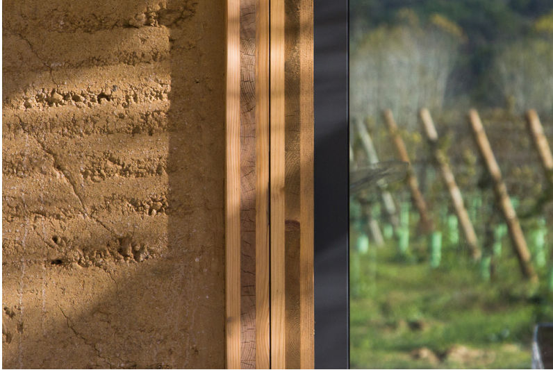
Abb. 44: Blaanc Architekten, Vineyard house, Montijo, Portugal, 2012, Fensterdetail
