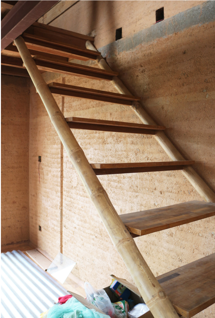
Abb.103: Abari, Dulikhel Learning Center, Dulikhel, Treppe aus Bambus, 10/2016
