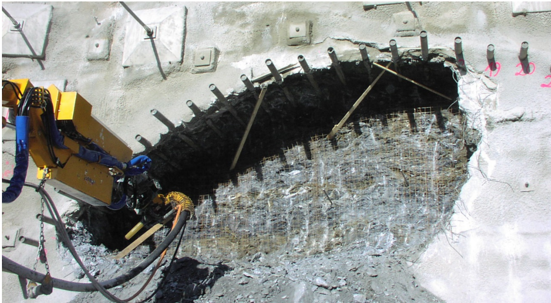
Figure 1 Portal pipe umbrella at Birgtunnel (Austria) [1]
