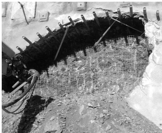
Figure 2. Pipe umbrella support at the Birgl tunnel portal (Austria)
