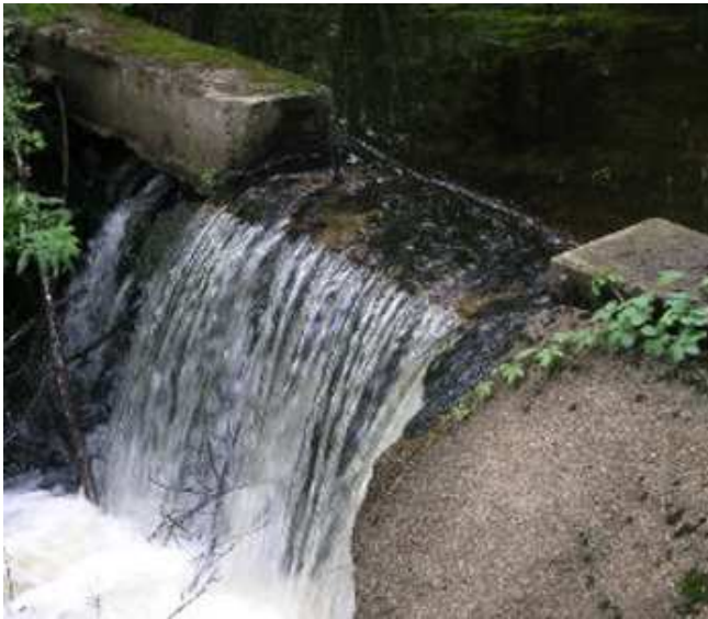
Figure 17 Example of a broad-crested weir (hydrocad, 2017)
