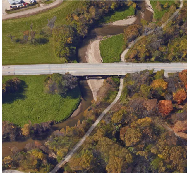
Figure 36 Satellite image of the gaging station „Walnut Creek at Des Moines” (google.maps, 2017)
