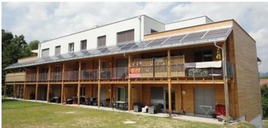
Figure 3-1 Building in Weiz (Hutter, 2016)
