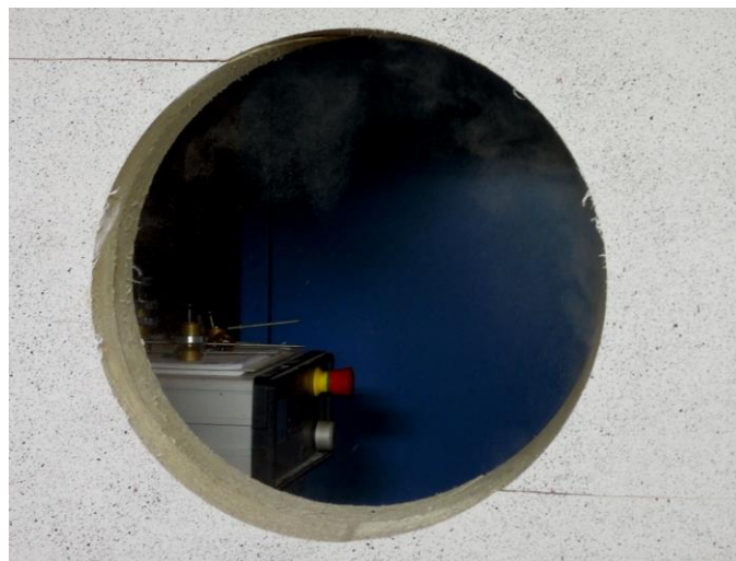
Figure B.18: Initial cracks on the upper left and lower right opening edge at 250 kN of test specimen D03
