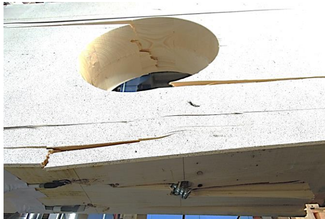
Figure B.27: Bending failure and cracks on the upper left opening edge of test specimen G01
