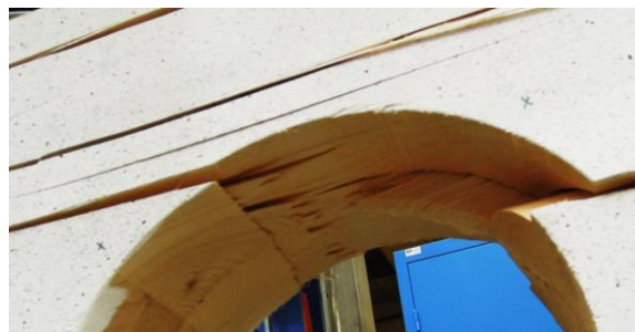
Figure B.35: Serrated initial crack on the upper left opening edge of test specimen H01
