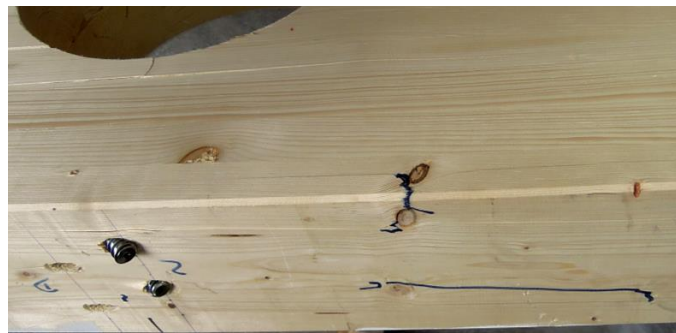
Figure B.20: Bending failure on the back and bottom side of the beam of test specimen D03
