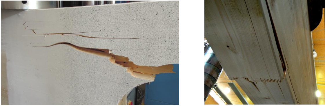
Figure B.11: Stepped propagation of the upper left crack on the opening on the beam front side (left); finger joints failure mixed with the bending failure in the gross cross section (right) of specimen C08
