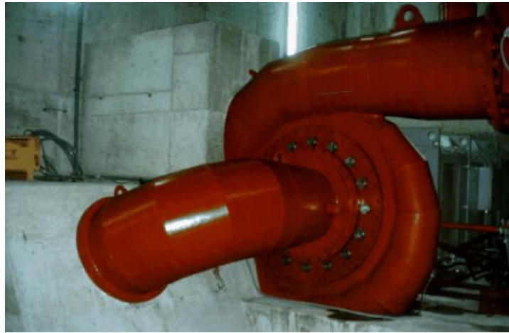
Figure 1-17: Horizontal axis Francis turbine (Source: [3a])
