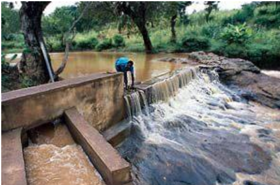
Figure 1-5: Intake with a weir to ensure the head for a small hydropower plant.
