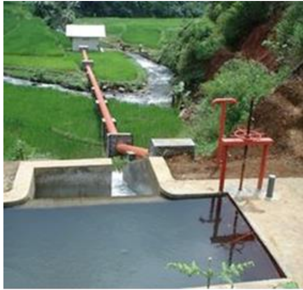
Figure 1-7: Intake, Penstock, Powerhouse
