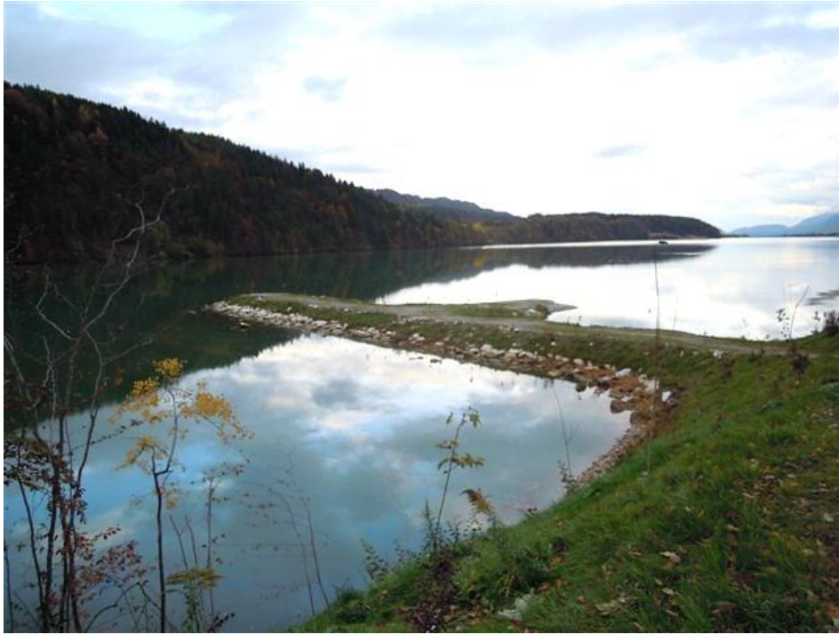
Figure 4.19: Photograph of the non-submerged groyne at cross section 600 (source: Verbund VHP)
