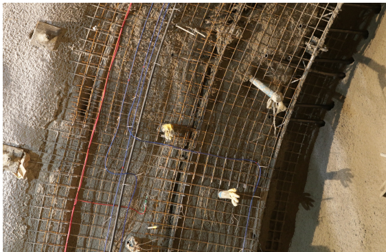
(c) Installed second layer, left side wall.
