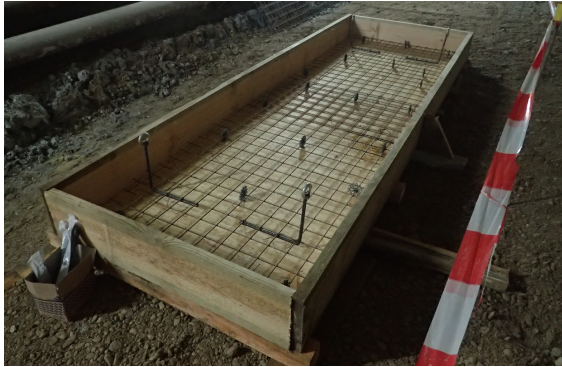
(a) Formwork for test slab.
