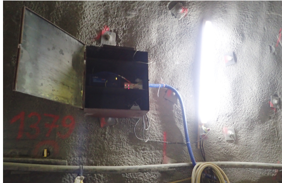
(a) Installed instrument box.
