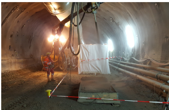
(e) Spraying of top layer shotcrete.
