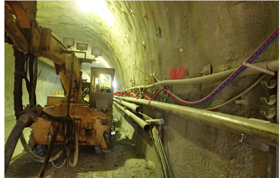
(b) Alignment of the supply cable.
