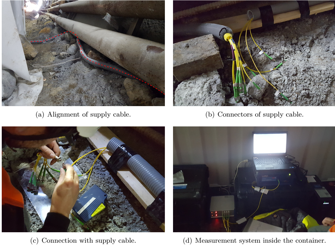
Figure 4.2: Measurements setup at the pre-test.
