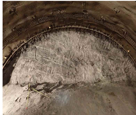
(b) Picture of face at chainage 1423.2 m.
