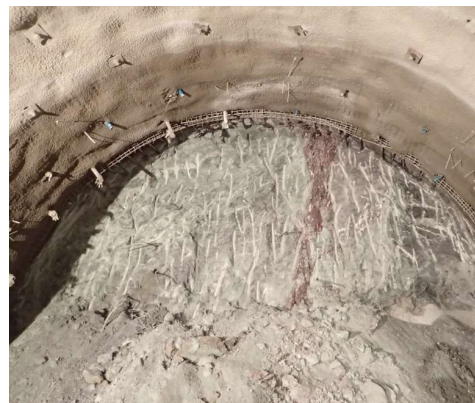
(f) Picture of face at chainage 1441.2 m.
