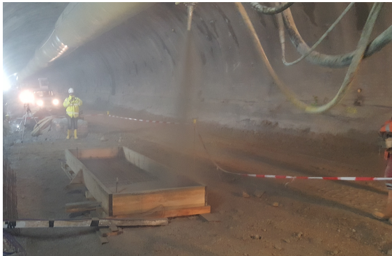
(c) Spraying of bottom layer shotcrete.
