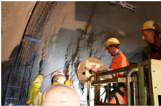
(a) Installation of first layer, left side wall.
