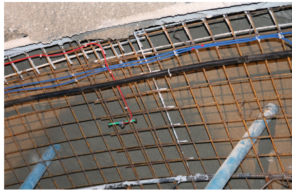
(b) First layer (with strain gage), crown.
